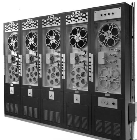
8-tracks of optical dubbers in late 1940s. The three right machines show loop cabinets for background effects such as rain. The right image shows how optical dubbers were simply updated with mag heads/electronics and continued to be used as 3-track mag dubbers. Optical dubbers like these, and even earlier machines from the late 1930s were still being used as mag machines in the 1970s due to the quality of their original construction. Photos: Endpoint museum collection.
