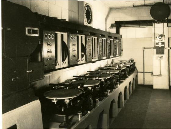
Examples of the earliest re-recording installations in the late 1920s and early 1930s. Left image shows 7 tracks of discs and one track of optical. Right image shows 4-tracks of optical dubbers. Additional machines are out of view in this image. Photos: Endpoint museum collection.
