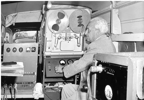
Example of remote production mag recording. Still often used within a sound truck like the earlier optical recording systems. Mag recording within the confines of a studio simply used the large mag machines shown in the previous section.
