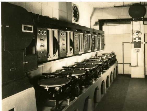
Examples of the earliest re-recording installations in the late 1920s and early 1930s. Left image shows seven tracks of discs and one track of optical. Right image shows four tracks of optical dubbers, which were modified projector soundheads. Additional machines are out of view in this image. Photos: Endpoint Museum collection.
