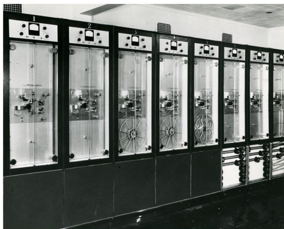
Left image shows eight tracks of optical dubbers in late 1940s. The three right machines include loop cabinets underneath for background effects such as rain. The right image shows how optical dubbers were simply updated with mag heads/electronics and continued to be used as three-track mag dubbers. Optical dubbers like these, and even earlier machines from the late 1930s were still being used as mag machines in the 1970s due to the quality of their original construction. Photos: Endpoint Museum collection.
