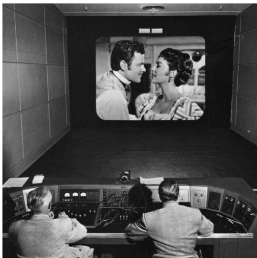
MGM 20-input re-recording console used for most mono films at MGM from early 1940s to 1970s. Only patched EQs on left and right side of console were present. Photo: Bison Archives
