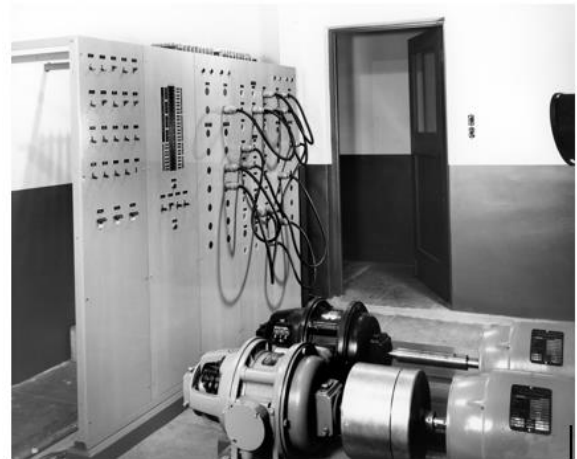
1950s-1970s Interlock generators and patch panel. Photo: Endpoint Museum collection
